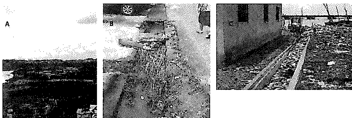
Fig 3a) Typical informal settlement, Lagos, Nigeria. 3b and c) Makoko, Lagos (b) Vegetation growing in a drainage channel due to lack of maintenance (c) drainage canal blocked with waste either carried there in surface water or deliberately placed there.
