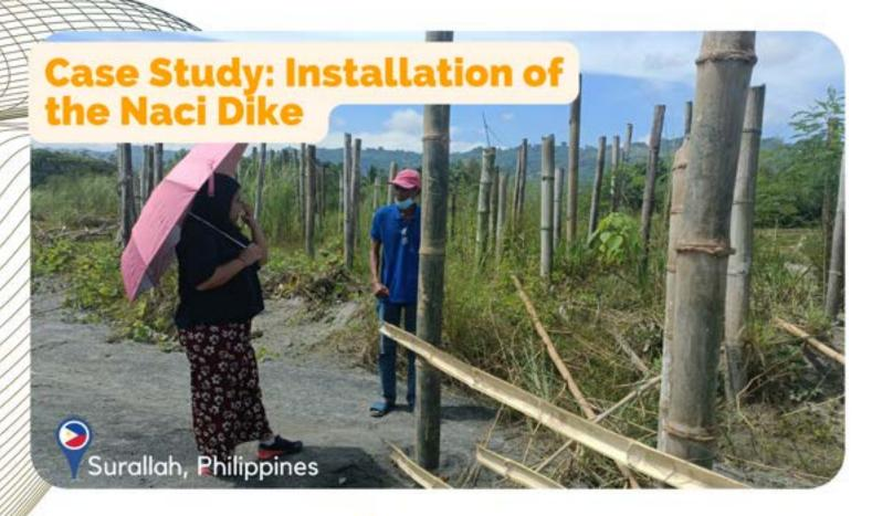
Building a dike made out of natural materials, to decrease the impact of flash floods of the Allah River. The dike will disintegrate over time and be replaced by planted vegetation.
